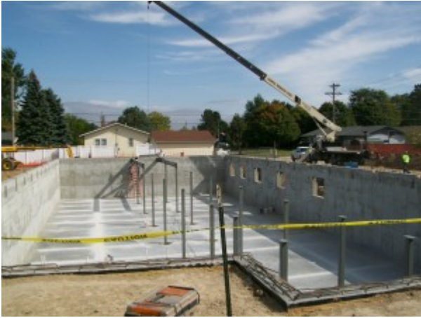
Steel reinforcements being erected for the main floor.
