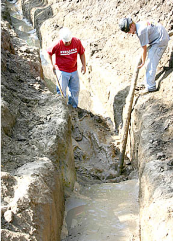
Sewer main work on Sixth Street.
