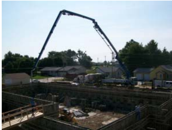
Foundation walls being poured
