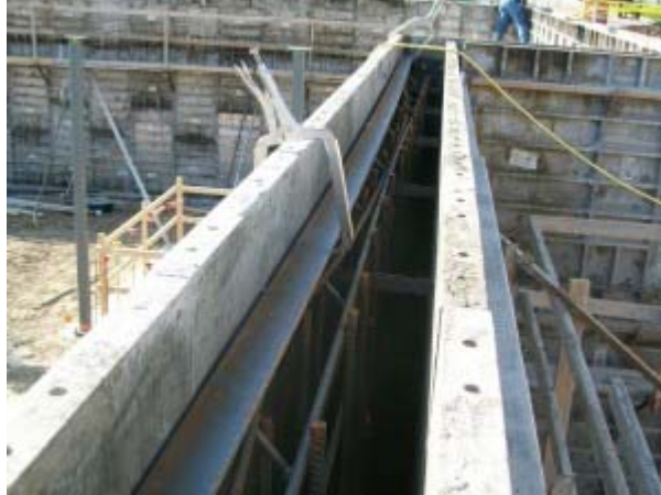
Embed angle being installed on west wall of basement
