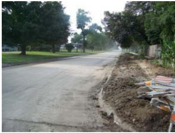
Sixth street after construction.
