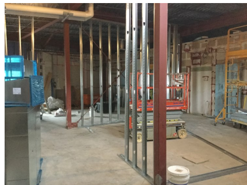
Interior framing in progress.
