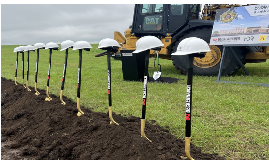
Ceremonial shovels used for the August 18th groundbreaking event. Following the event, crews prepare the site for the beginning of construction.
