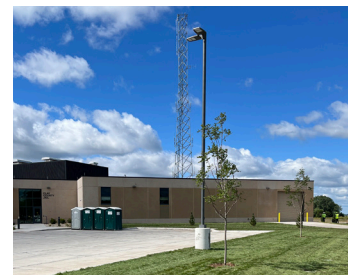
The new communication tower enhances emergency response and connectivity for Clay County.
