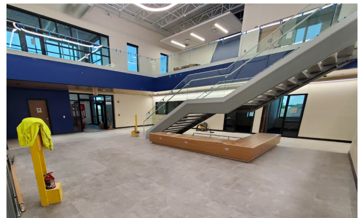
The new lobby area is designed to inspire, featuring terrazzo stair treads, glass handrails, and wood plank ceilings.
