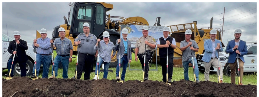
Joe Beckenhauer joined community leaders, county officials, and law enforcement representatives as they broke ground at the ceremony.
