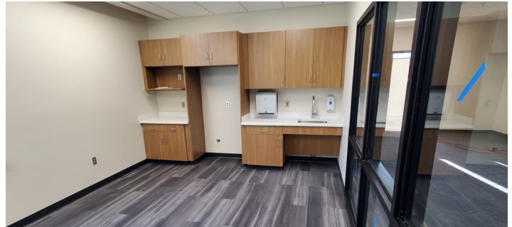
The John N. Harms Center Health Sciences Building project will create a new and improved learning environment for the next generation of nurses, healthcare providers and educators.
