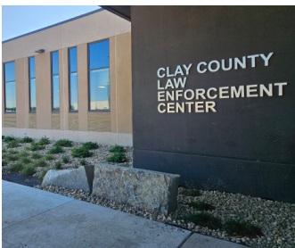
The entrance to the building complete with new signage and landscaping.
